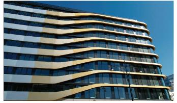
Hueck's unitized façade design has been successfully used in international projects for many years and undergoes continuous further development, amendment and optimization of insulation properties. Based on this experience, Hueck's project engineers have developed a standard series: the highly insulated unitized façade construction **Trigon Unit L**.
